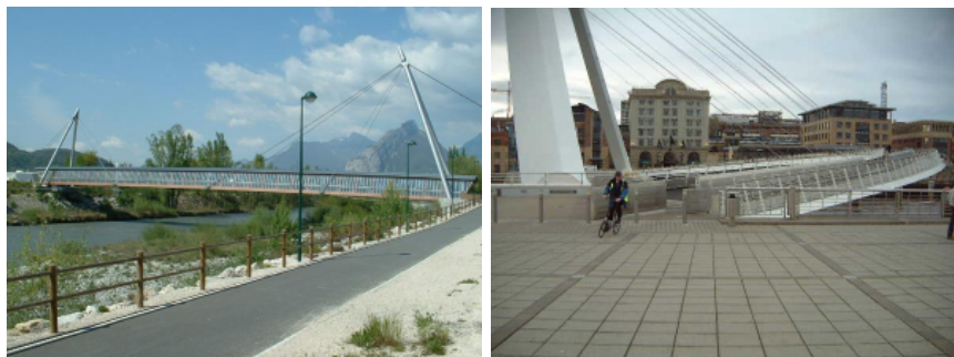
Cycle bridges at Grenoble, FR and Newcastle, UK
